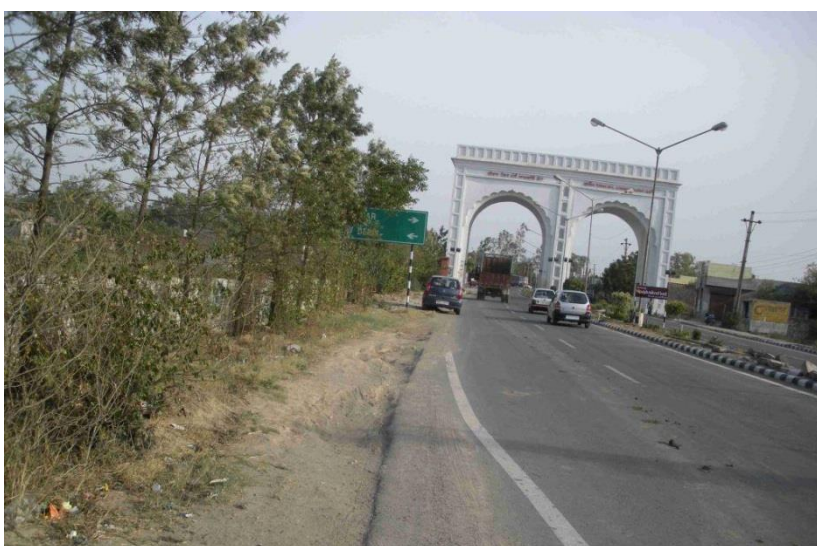
Figure 7. Shoulder Maintenance & Sign Visibility – Non Conformance
