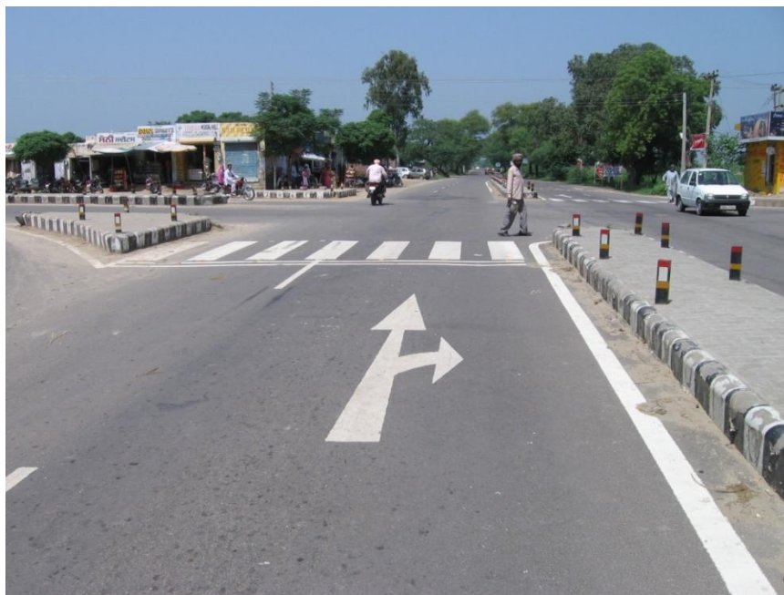
Figure 20. Conforming Pavement Marking - Intersection – Pedestrian Crossing
