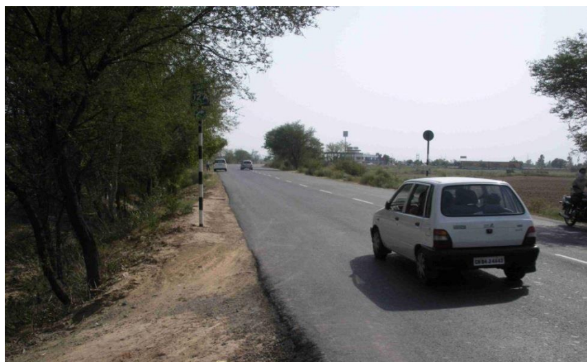
Figure 15. Vegetation Control (General) Non Conformance (Sign Obscured) & Shoulder Maintenance Non Conformance (Edge of Seal Drop Off)
