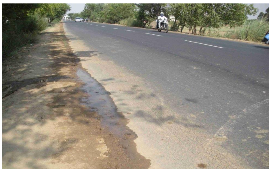
Figure 9. Ponding and Shoulder Maintenance – Non Conformance
