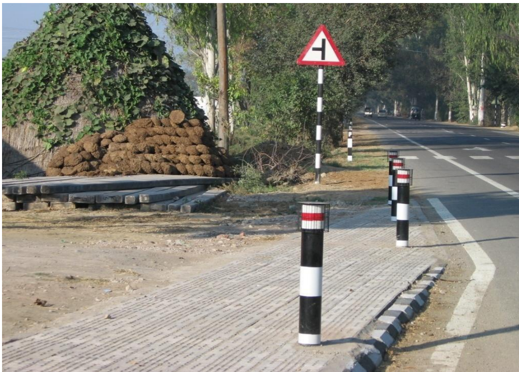
Figure 22. Conforming Delineators and Signage
