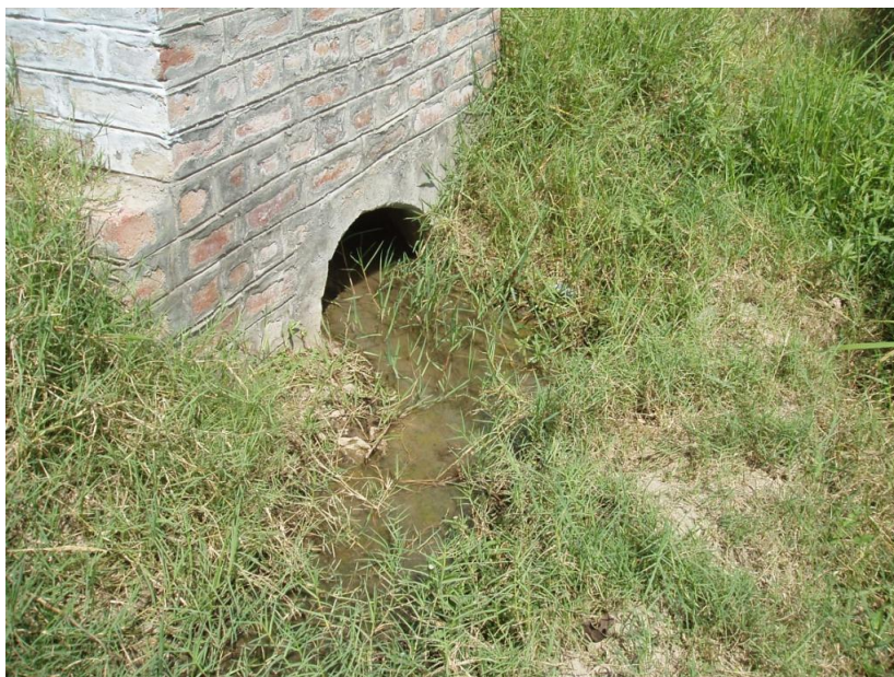
Figure 10. Drainage Culverts –Non Conformance (Vegetation & Silt)
