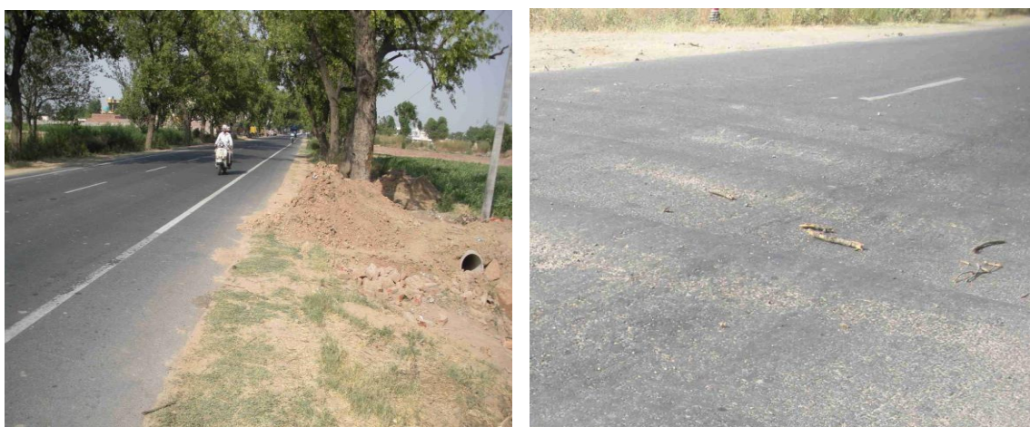
Figure 13. Obstructions on the Pavement and Shoulder Non-Conforming (Debris Accumulated on the Shoulder Spilling on to the Pavement)
