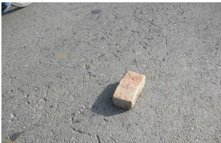
Figure 5. Surface Cracking (Brick Provided for Scale) – Non Conformance
