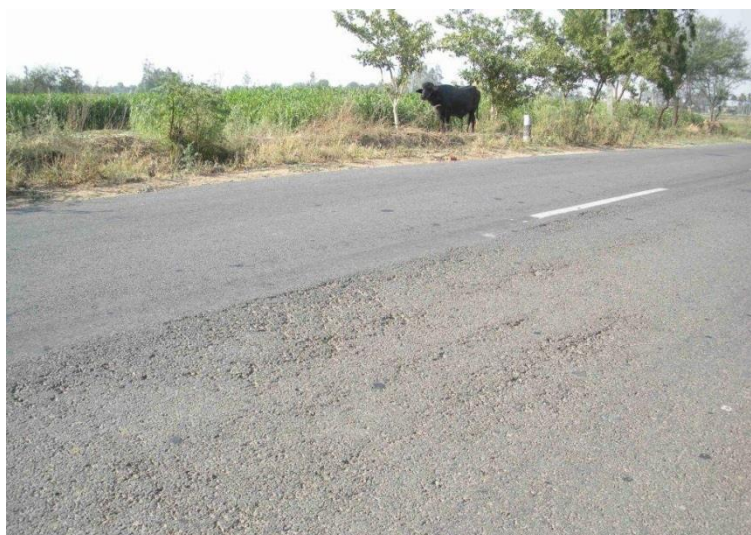
Figure 4. Surface Ravelling - Non Conformance
