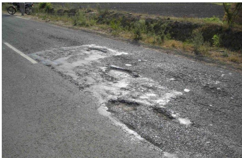
Figure 6.Surface Pot Holes – Non Conformance
