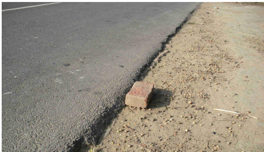
Figure 8. Shoulder Maintenance – Non Conformance (Brick Provided For Scale)
