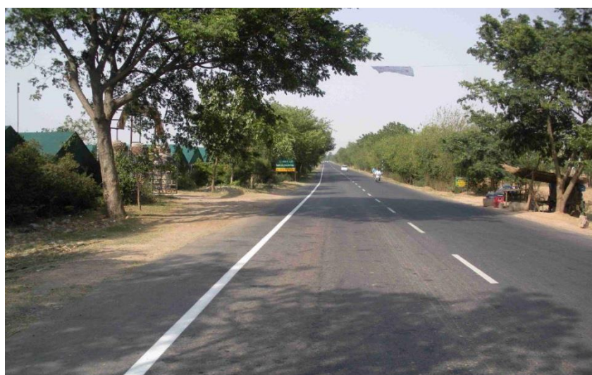
Figure 19. Pavement Marking Non Conformance (Edgeline marked only on one side)
