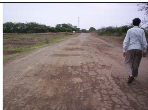
Block cracking Km 14+775 to14+875 (SH-160) Padra-Karjan roda
